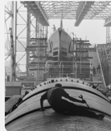
Man working on Hull of U.S. Submarine Connecticut, August 1943
